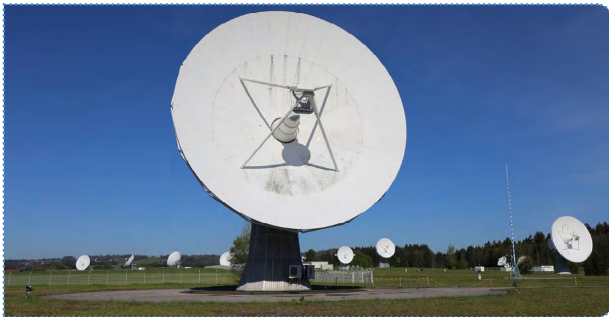
15-metre S-band antenna at the DLR site in Weilheim. DLR's German Space Operations Center (GSOC) will support the Artemis II mission using the ground station in Weilheim. It will receive signals from Orion and track the spacecraft's flight around the Moon from Earth. Credit: © DLR (CC BY-NC-ND 3.0)
